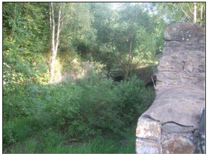
The Canal Tunnel Entrances
